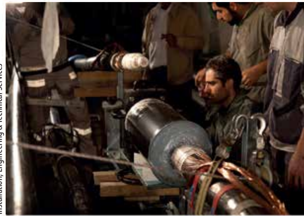
Installation, Engineering & Technical Services
