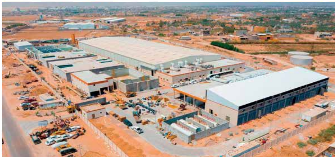
Basra Desalination Plant - EPC Project
