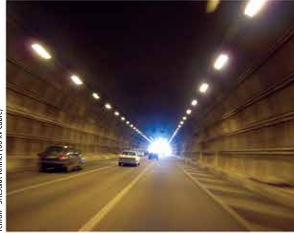
Tehran - SResalat Tunnel (66 KV Cable)
